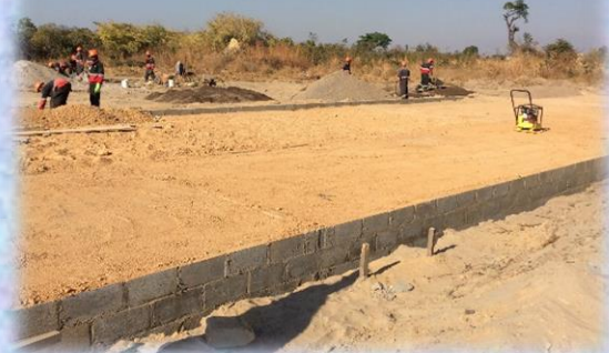
Preparing the classroom module slab
